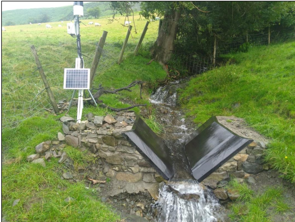
Figure 7-1: The Canada Wood flume to the North of Sedbergh.
