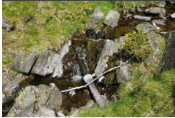
Figure 86: FID33 - Pipe crossing Settlebeck Gill, facing north west.
