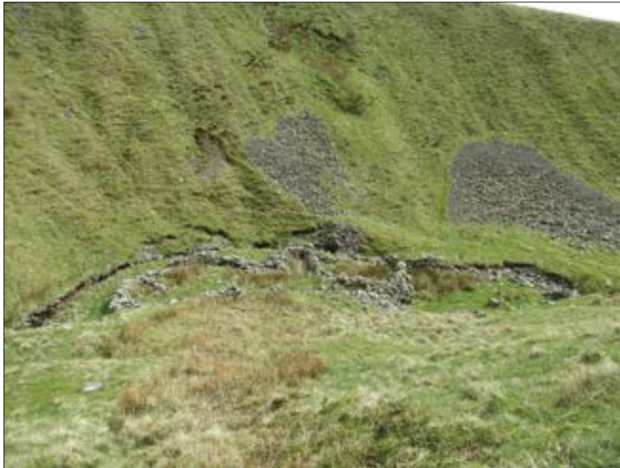
Figure 21: Washfold in Ashbeck Gill, MYD60674 (FID3), known as Ashbeck Fold. The remains of the dam with a partly collapsed revetment wall is visible centre right, behind the fold.
