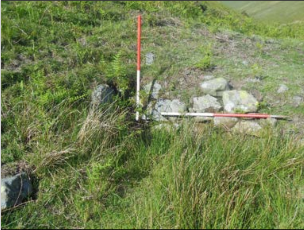
Figure 139: FID96 - A short section of stone wall located on the north side of Crosdale Beck built into the hillside.
