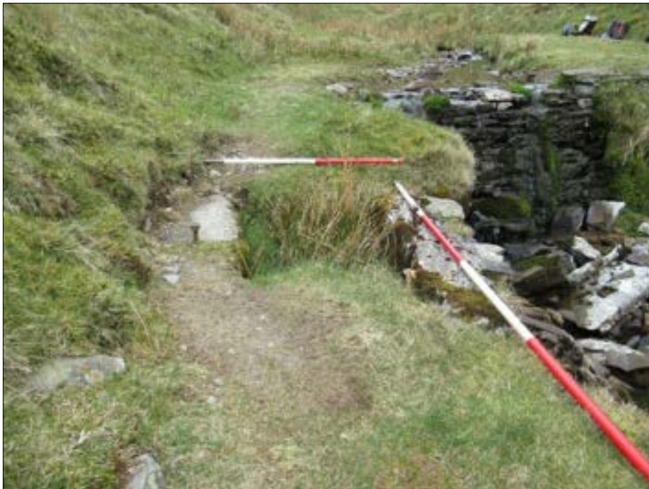
Figure 66: FID2 - Chamber and pipe track with the revetment wall top also visible to the right, with the dam (FID1) in the background, Ashbeck Gill.
