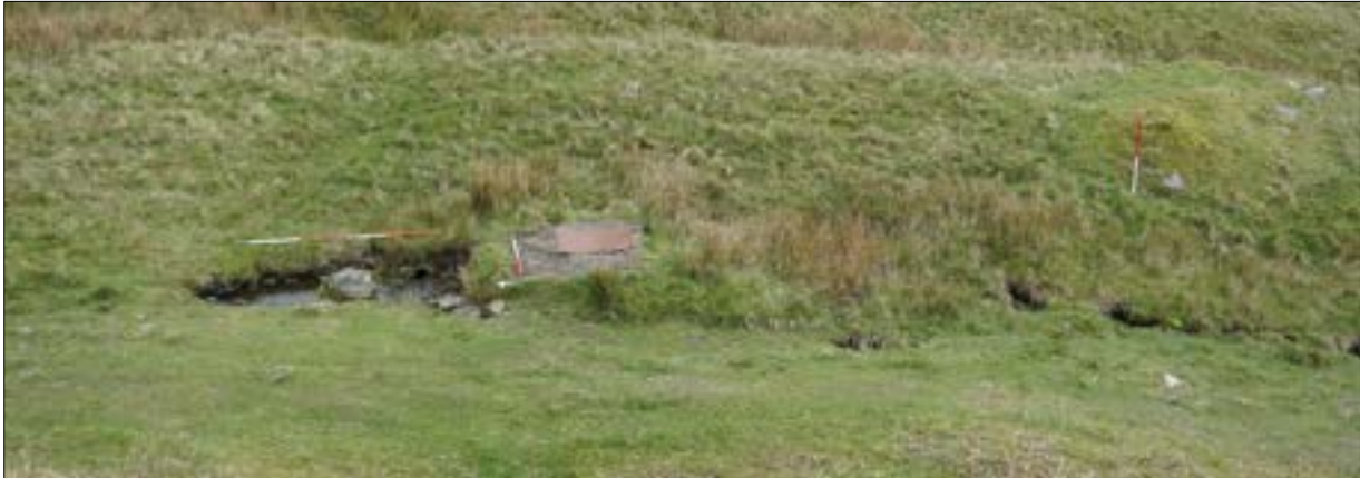
Figure 31: FID25 – A concrete chamber, pond and spoil heap (behind upright ranging rod, right side), west side of Settlebeck Gill.
