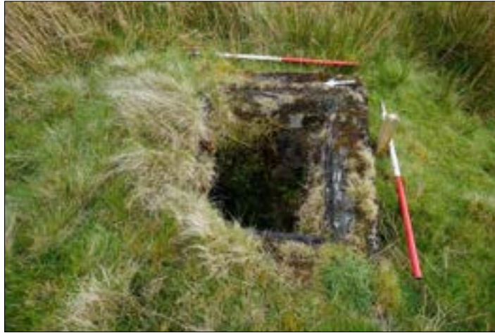
Figure 83: FID28 - Concrete chamber forming part of the former water supply for Sedbergh Town, head of Settlebeck Gill, facing east.
