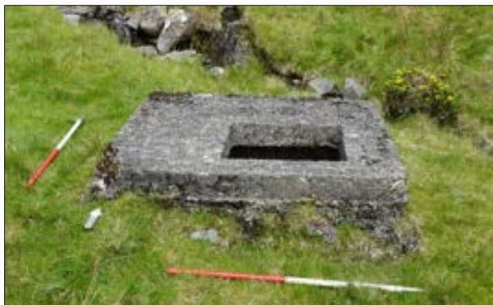
Figure 85: FID32 - Concrete chamber forming part of the former Sedbergh Town water supply system, Settlebeck Gill, facing north.
