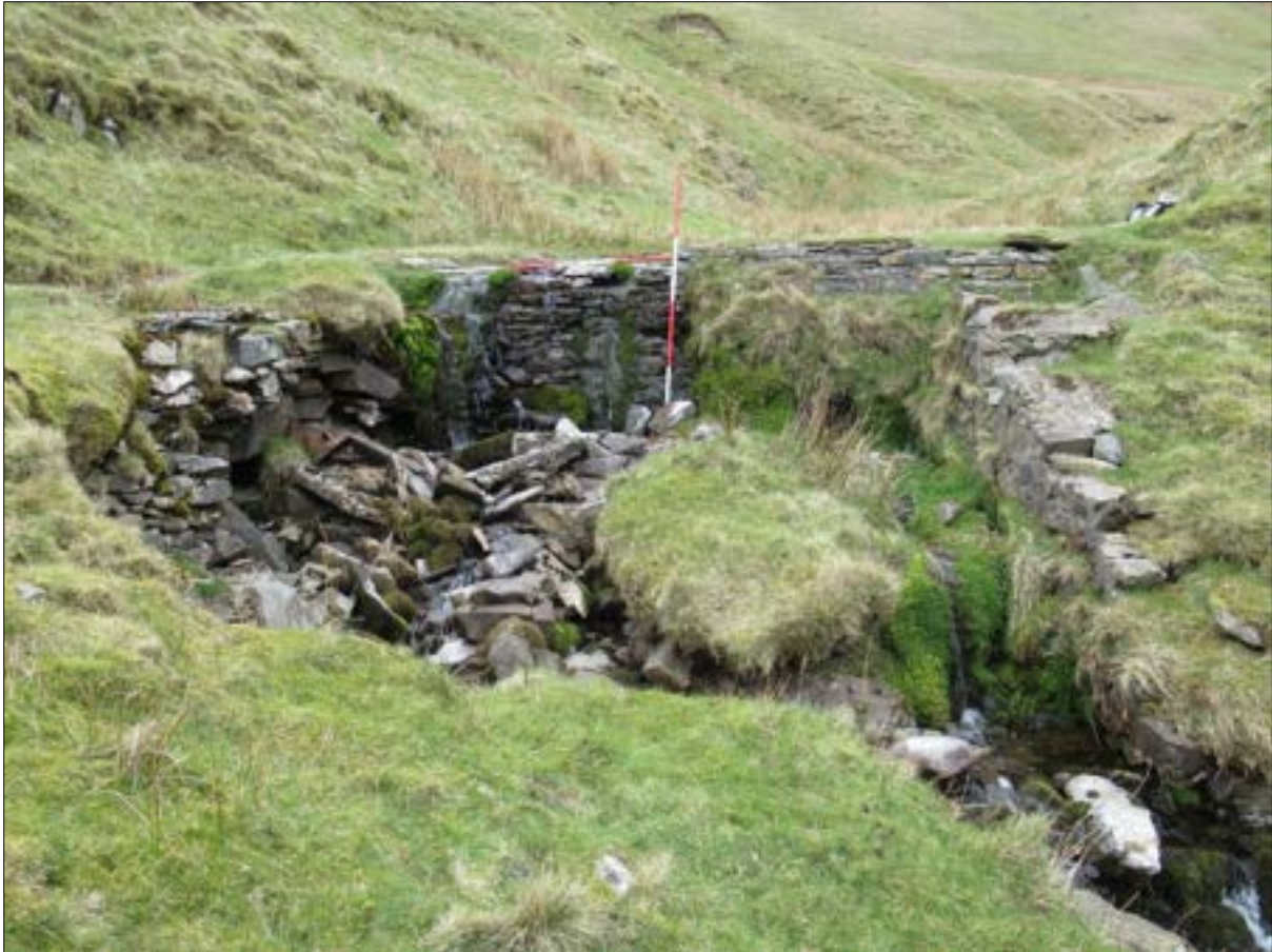
Figure 25: FID1 - Dam with infilled reservoir behind in Ashbeck Gill, formerly associated with the historic water supply system for Sedbergh Town.
