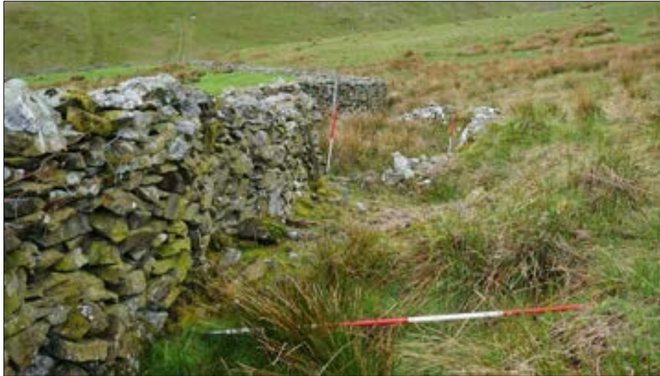
Figure 77: FID20 (MYD50570) – Oval sheepfold with annex at its eastern end (foreground), built into a bulge in the boundary wall.
