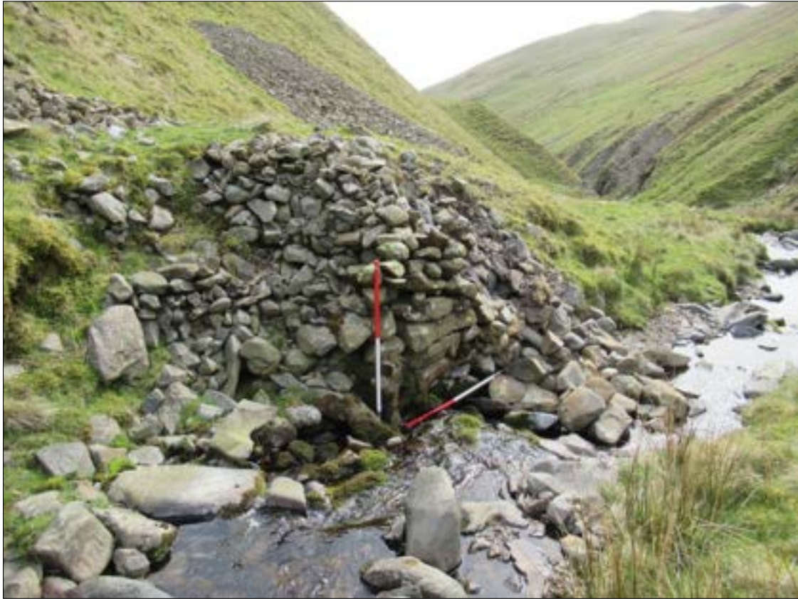
Figure 23: FID4 – former dam with revetment wall adjacent to FID3, showing the location of a former sheepwash.
