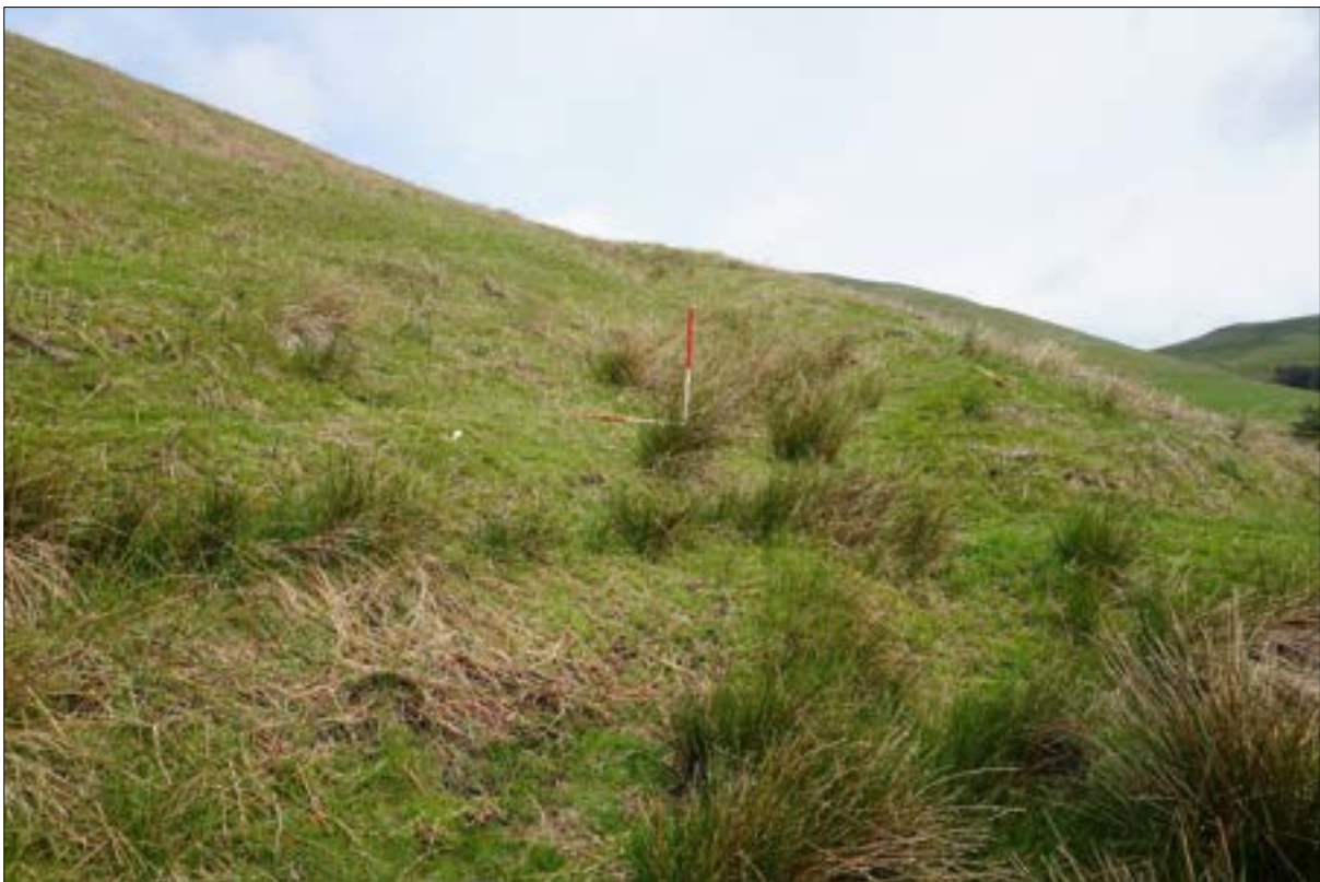
Figure 27: FID38 - bank with ditch on its western side, Crook.
