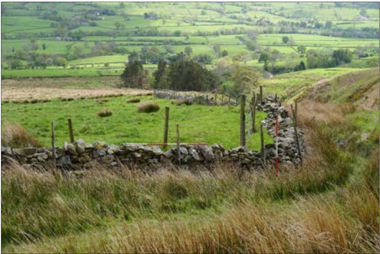
Figure 20: Bank, forming part of FID23, just visible on the south side of the common boundary wall.
