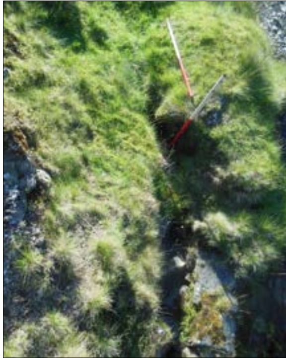
Figure 141: FID97 – View of the end of the leat and the structure (right hand side) on the south side of Crosdale Beck, located next to the weir shown in figure 140.
