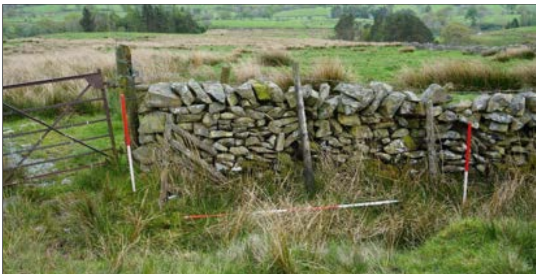
Figure 79: FID21 - Boundary wall, facing south east.
