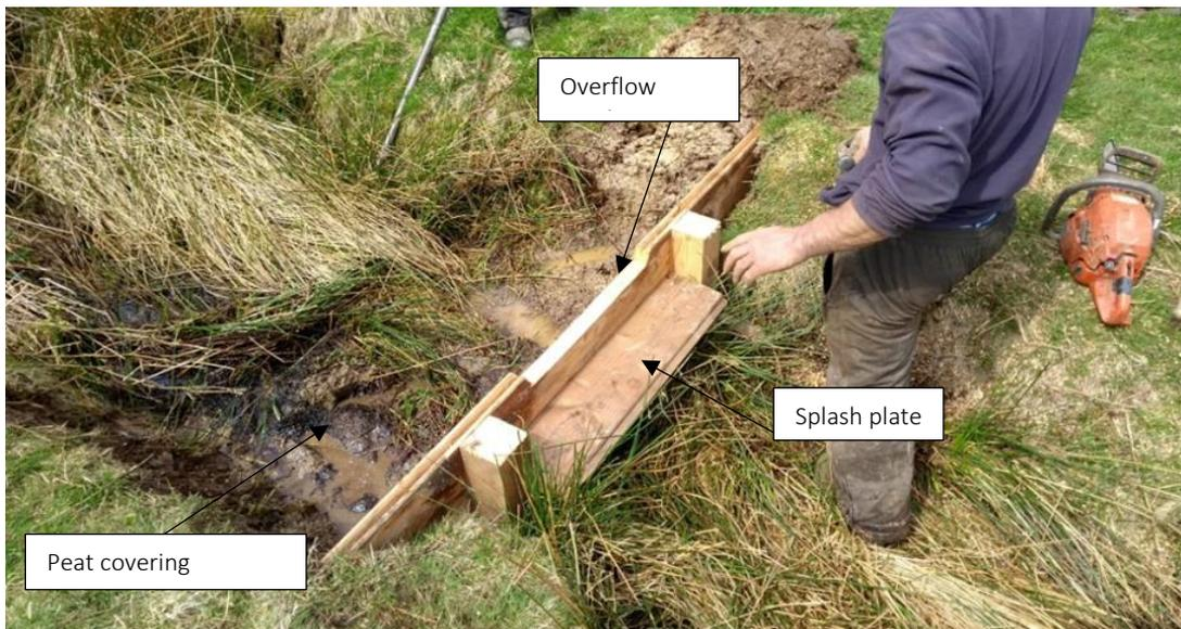
Figure 4: Woody dam block being installed showing downstream splash plate, overflow notch and upstream peat covering
